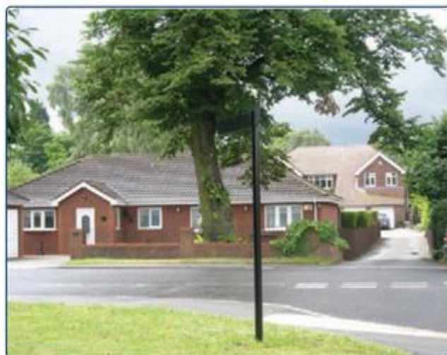
Figure 24 - Backland properties should not be larger in height, massing, scale and volume than the host dwelling, as in this example where the property is highly visible behind the host bungalow and creates overlooking from first floor windows
