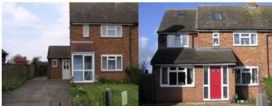
Figure 11 - Before and after photographs showing a sympathetic side / front extension which is well proportioned in relation to the host
