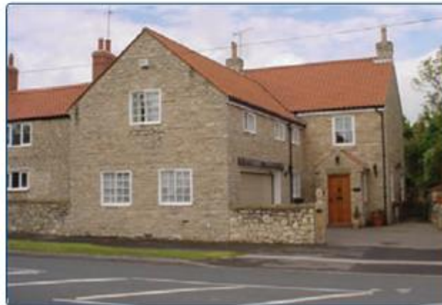
Figure 22 - Infill in conservation areas and other areas with character require an in depth appreciation of the character and qualities of the area, so the new buildings sit comfortably in it. The top example is appropriate in terms of its form, but the materials (especially fencing) are at odds with the prevalent stone used in the conservation area. The bottom example is better in terms of material and detailing
