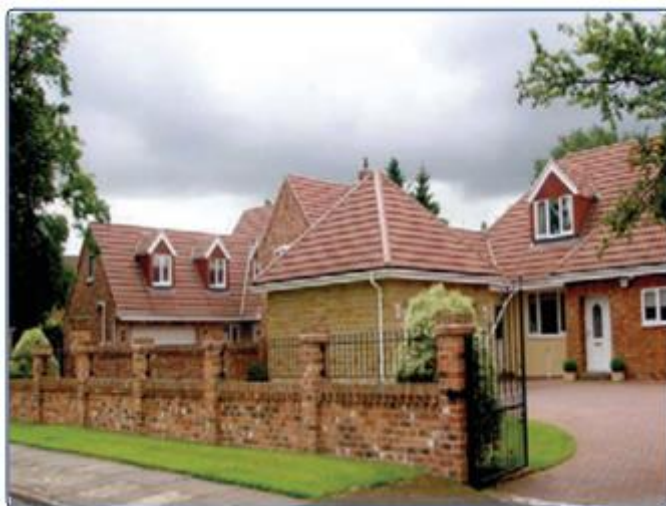
Figure 18 - Insensitive positioning of this garage block to the front of the property has had a negative impact on the character of the street by introducing a prominent structure in otherwise open front gardens
