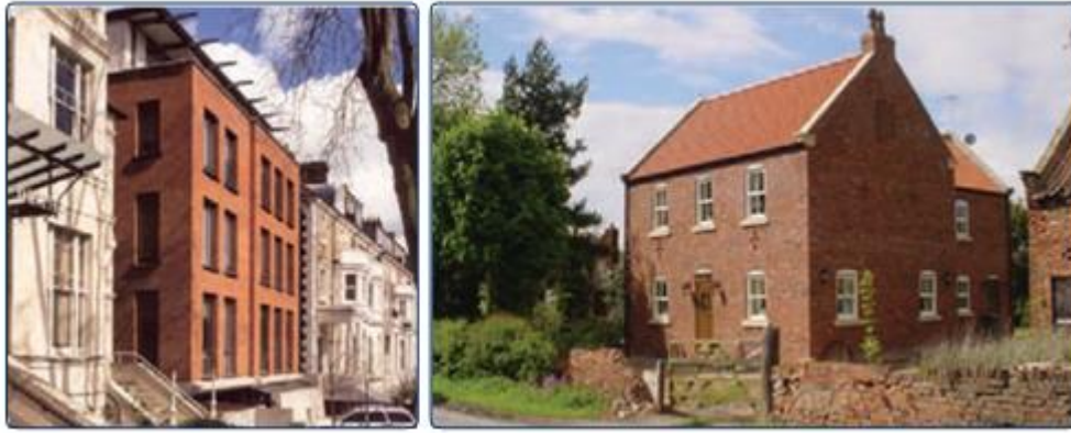
Figure 29 - Left image: the contemporary architectural style contrasts with the prevailing style to create variety within the streetscene. Whilst architecturally different, the infill development conforms to the general plot width, building height and building line of the street (from 'Building in Context', English Heritage & CABE, 2001); Right image: this infill development is sensitive to the traditional, semi-rural character of the street in terms of its visual separation and form. It follows the established building line and features restrained fenestration and detailing appropriate to this character.
