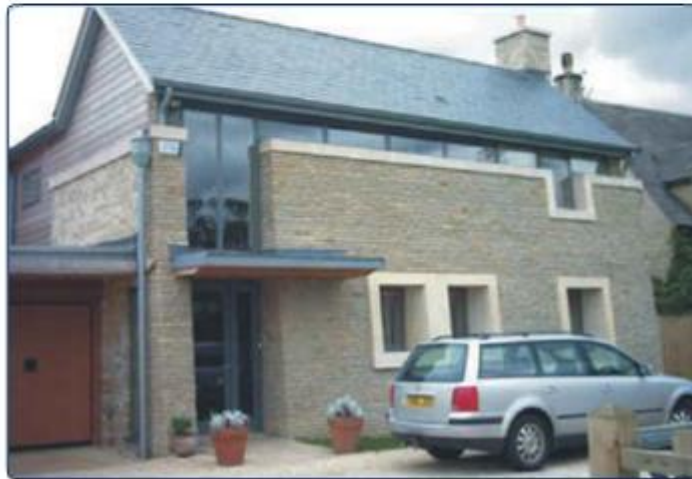
Figure 1 – Top: sometimes in historically sensitive areas it may be better to reflect the existing vernacular as this new development does successfully; Bottom: contemporary interpretation of vernacular design is desirable and will be supported where it will make a positive contribution to the area.
